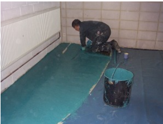
Ecoscreed Deco - Verde screed application
